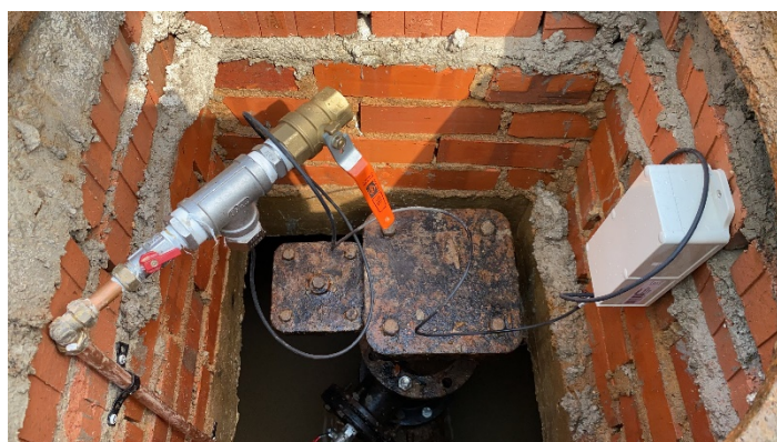
Aquarius Spectrum's Acoustic Hydrophone Sensor Installation
